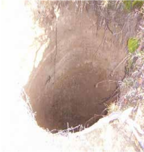
Very old and uncovered vertical mining works in Gumnishtë
